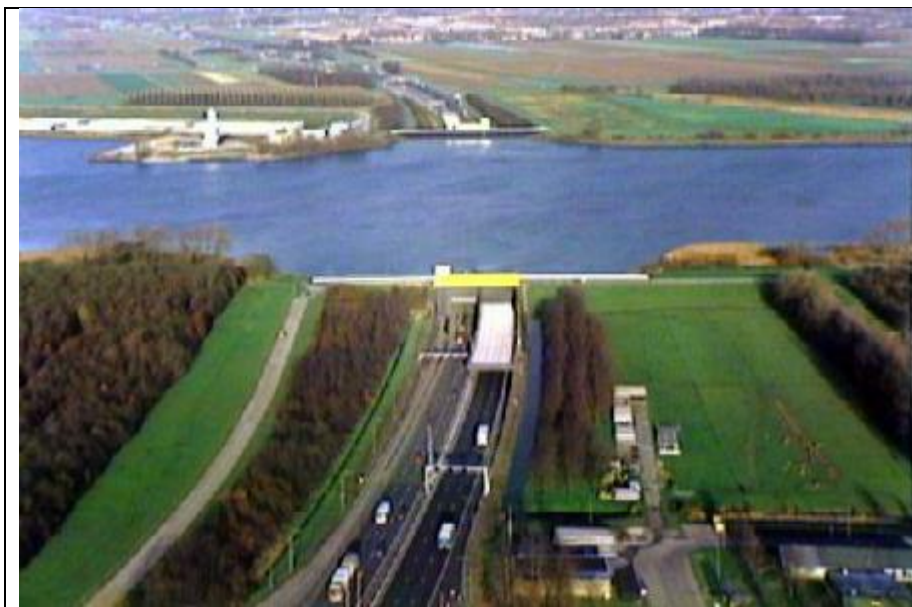
Heinenoordtunnel 1.064 m 1991, Netherlands
