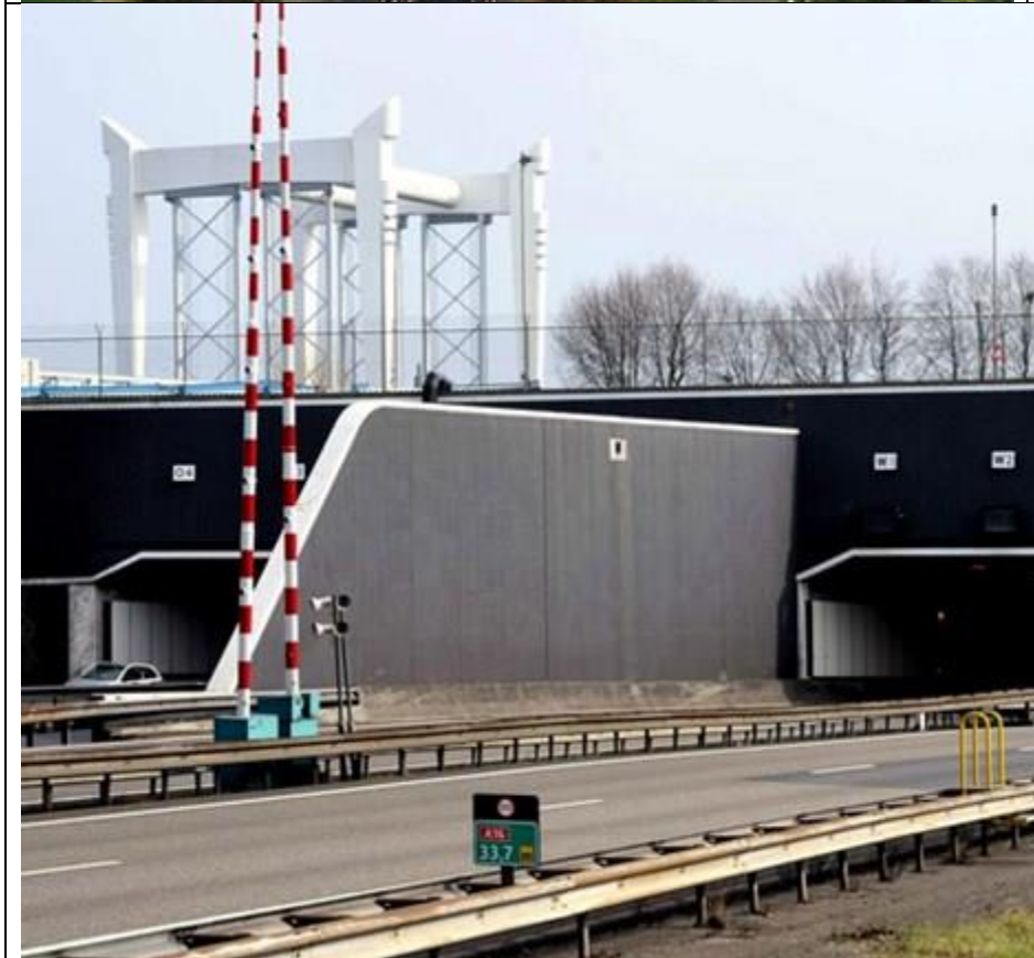
Drechtunnel 823m 1991, Netherlands
