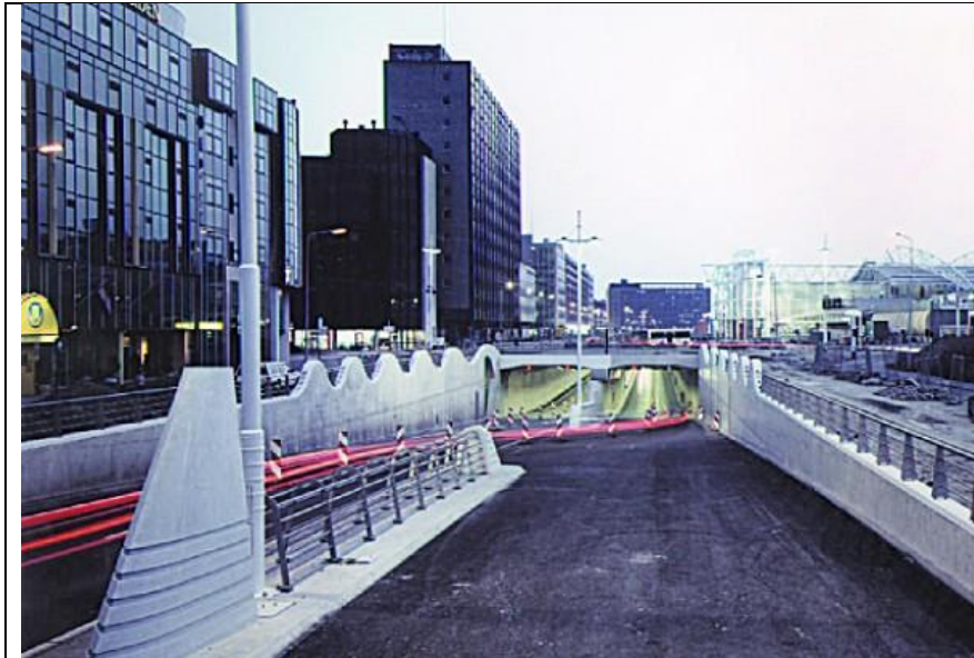
Stationsplein tunnel 500 m
